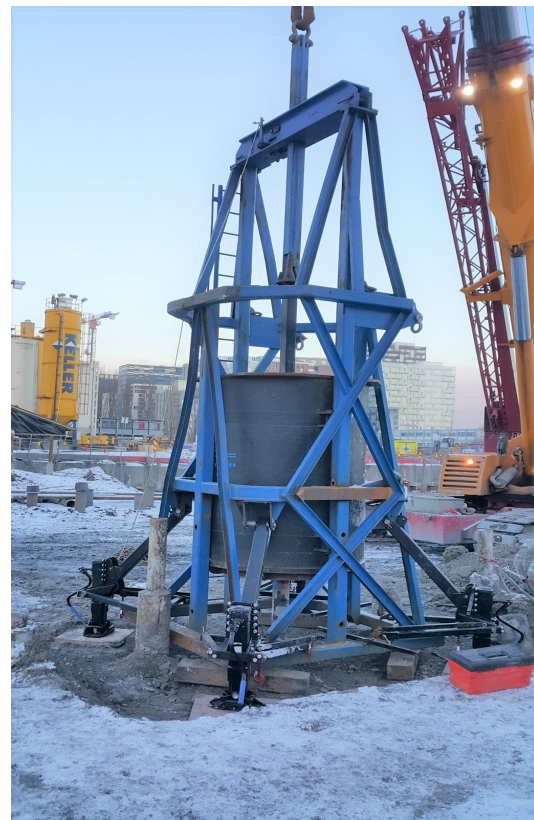
PP12 standing on ground (G)
