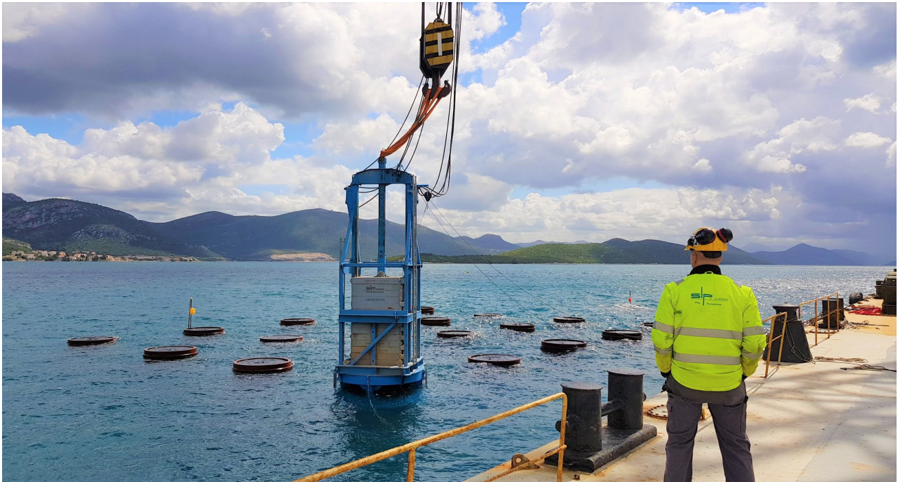
Dynamic load test (DLT) with PP54 ; pile diameter=2000mm; location: Bridge Pelješac, CRO
